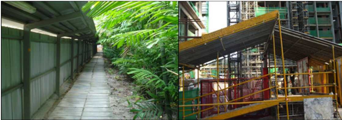
Photo 2.5a: Covered walkways around the perimeter as well as within the site provides protection and shelter.
