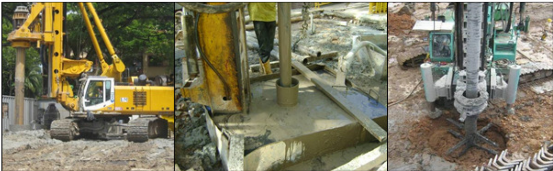
Photo 2.6g: Correct choice of piling system will mitigate noise and vibration felt by surrounding residents.
