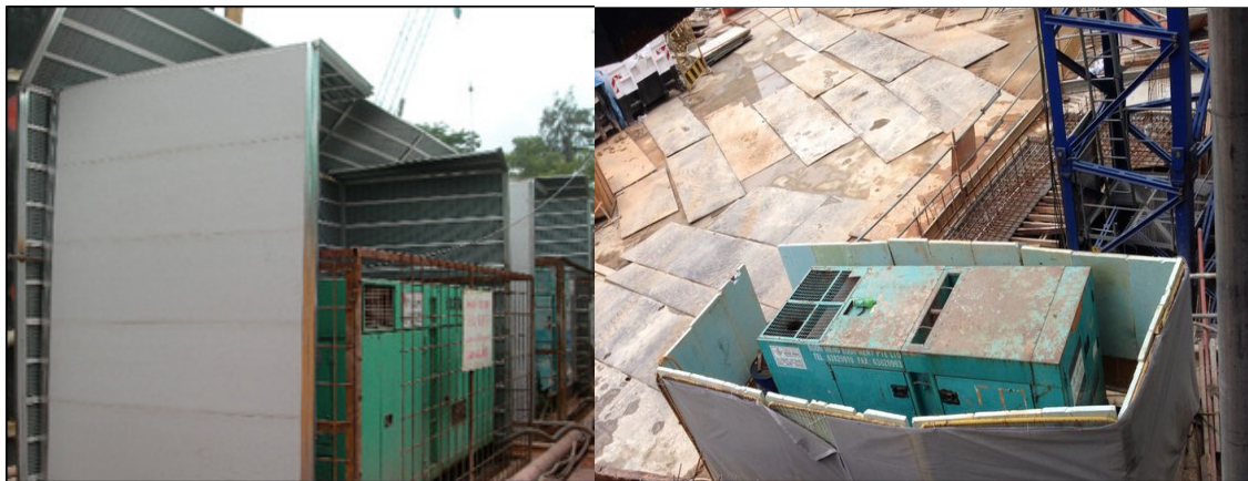
Photo 2.6b: Noise barrier panels around generators and machinery help to reduce the noise transmitted.
