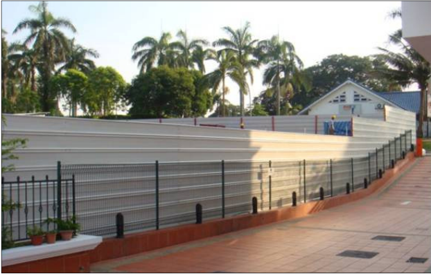
Photo 2.5c: Hoardings are maintained in good and clean condition through regular maintenance.
