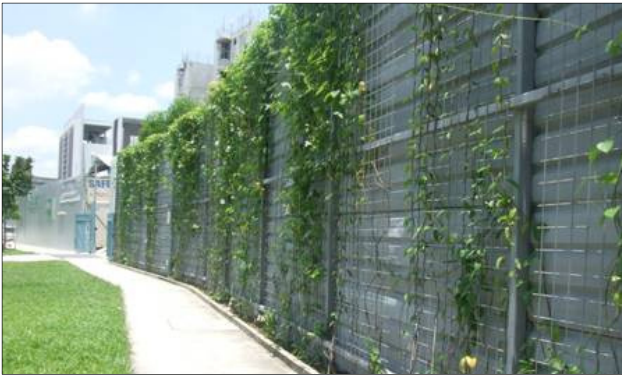
Photo 2.5d: Hoardings with vertical greens can look pleasing to the public.
