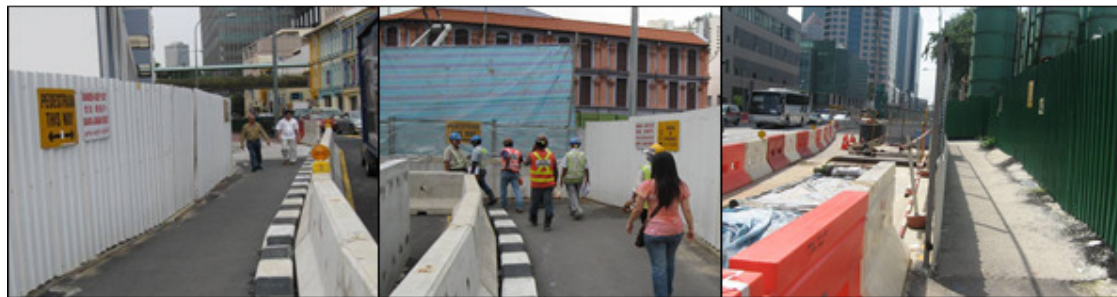
Photo 2.5e: Some examples of passageways provided around construction site.
