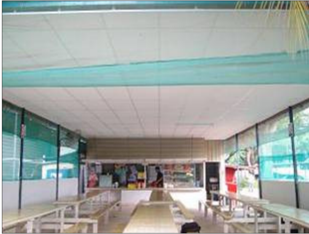
Photo 3.1c: Netting and false ceiling for canteen area ensure staff and workers can rest and eat in a cooler and dust free environment.
