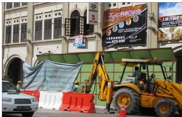
Photo 2.6c: Use of movable noise barriers can also reduce the noise transmitted from machinery.
