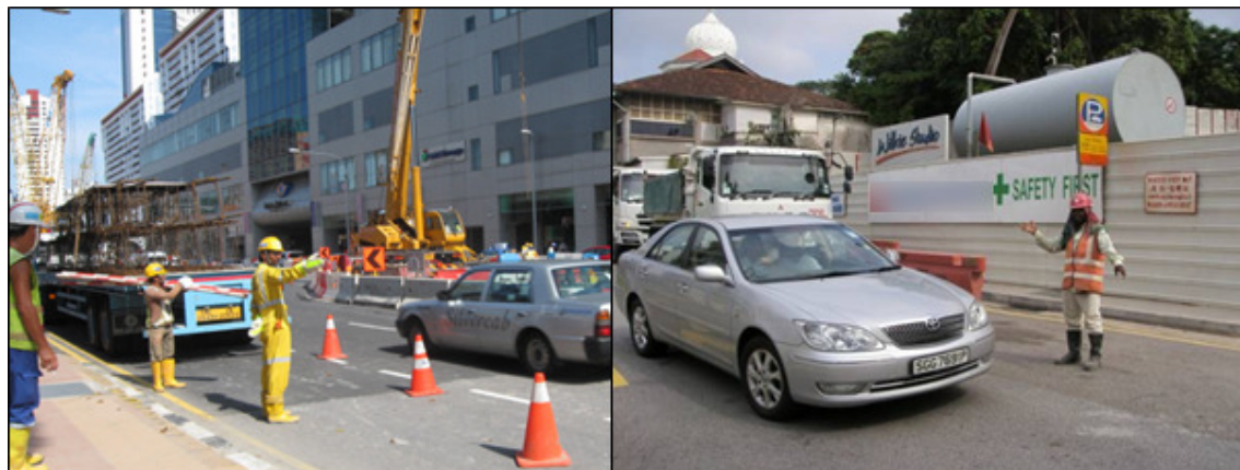
Photo 2.4d: The traffic controller guides traffic during concreting operations or materials delivery.
