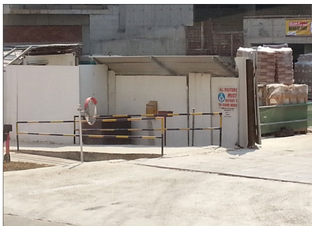
Photo 2.4e: A traffic mirror can be used to show blind spot.
