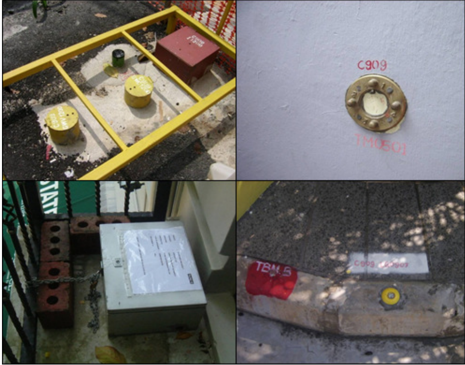
Photo 2.5f: Comprehensive monitoring of surrounding buildings can be done through the use of inclinometers, tilt meters, vibration meters and settlement markers.
