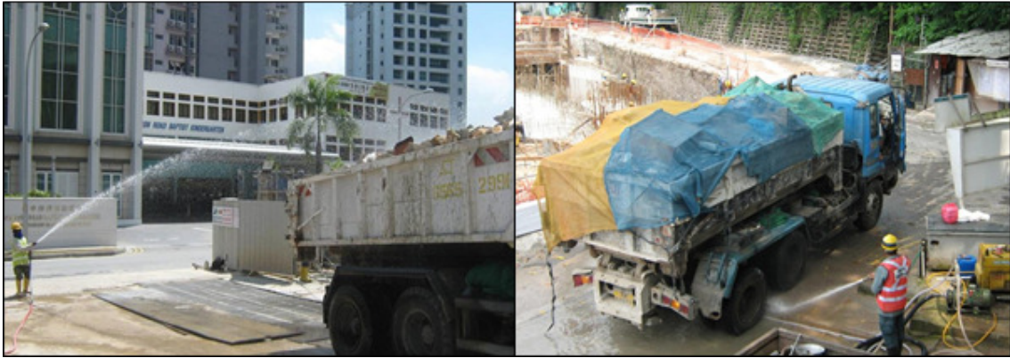
Photo 2.3e: Spray water to dampen dust generating materials and cover them properly during transportation.
