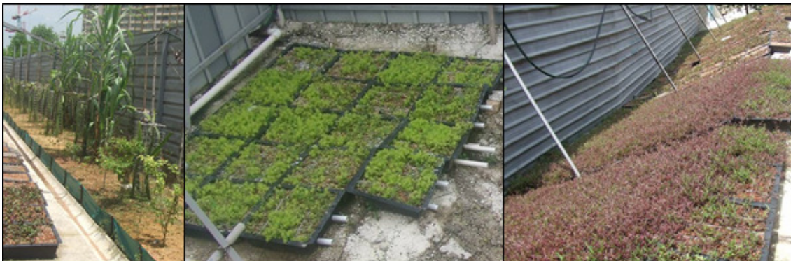
Photo 3.1b: Where space is available, plants and flowers can be planted extensively to beautify the site environment. These plants can also double up as erosion control measures to enhance the quality of water discharged out of the site.
