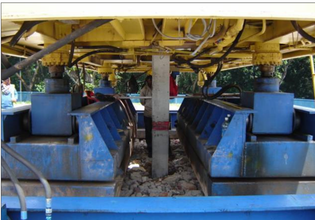
Photo 2.6f: Silent jack in piles greatly reduce noise and vibration produced.
