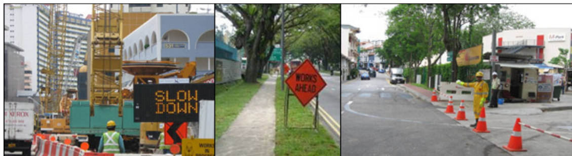
Photo 2.4g: Variable message sign (VMS) system complements role of traffic controller and usage of signages. This tool helps to minimize inconvenience to the public.
