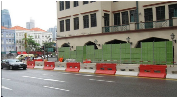
Photo 3.2a: Movable noise barrier can be used extensively at various locations where construction works are ongoing. It is an effective and easy way to reduce noise transmission to the public. There is also cost saving as no permanent noise barrier needs to be installed.
