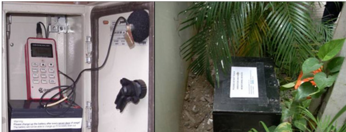
Photo 2.6h: Noise and vibration meters are installed for monitoring purpose.
