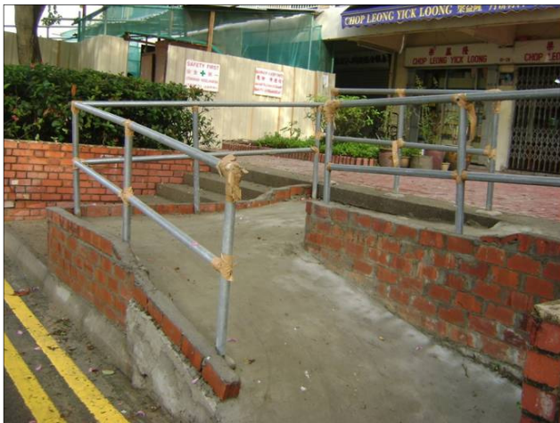
Photo 2.4b A temporary ramp helps pedestrians at a walkway affected by construction works.
