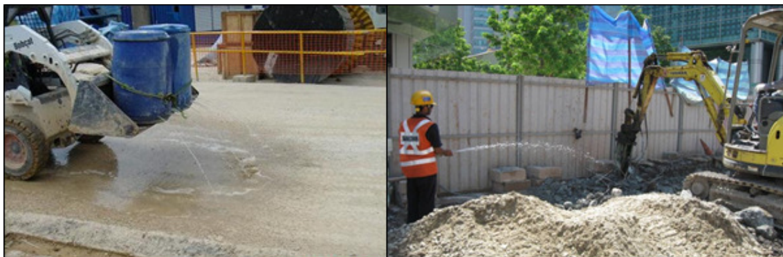
Photo 2.3d: Spraying water on site access roads and during hacking works will reduce dust generation. This is especially effective during dry days.
