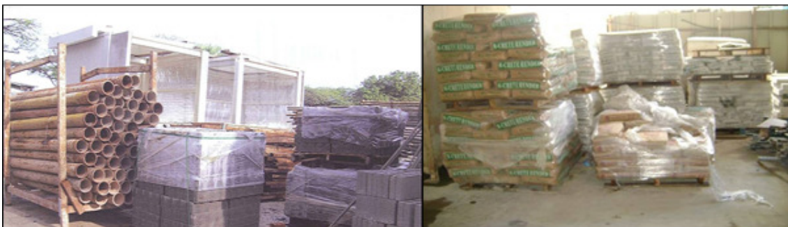
Photo 2.3a: Designated storage spaces allow materials to be properly stored on site.
