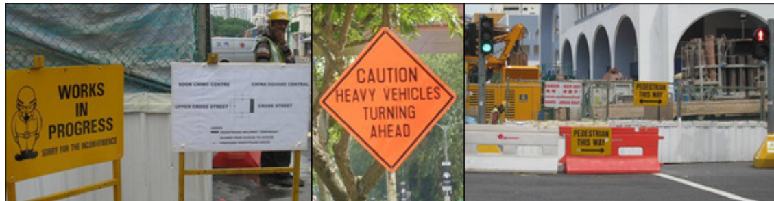
Photo 2.4f: Some examples of good signages around the construction site.
