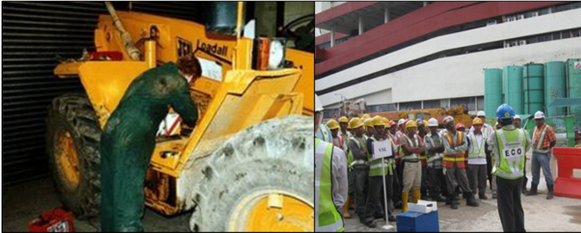
Photo 2.6d: Machinery is regularly maintained and workers are properly trained to handle them.
