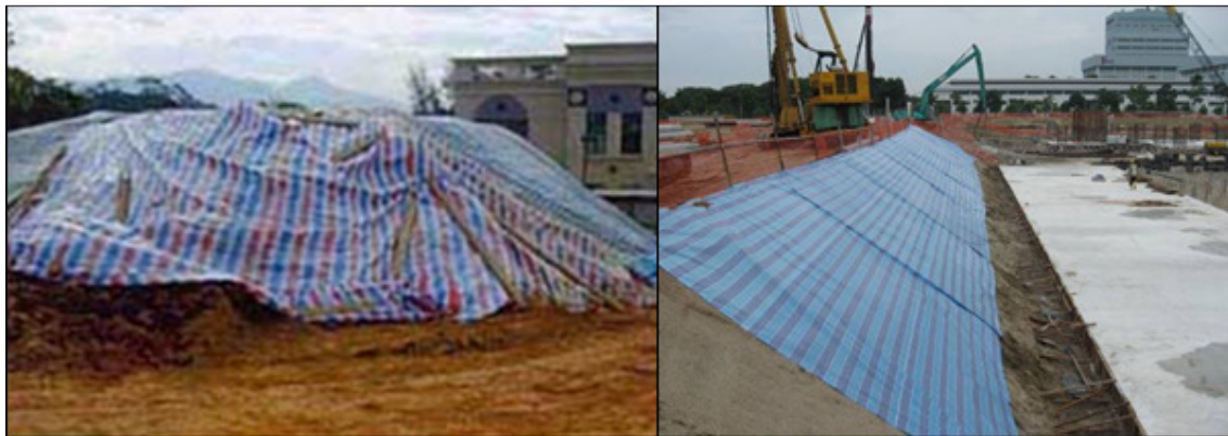
Photo 2.3c: Covering stock piles with sheets help to mitigate dust generation on site.
