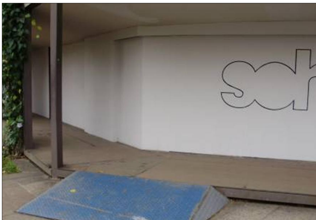
Photo 2.4c: A temporary ramp besides site hoardings is also useful to public users.
