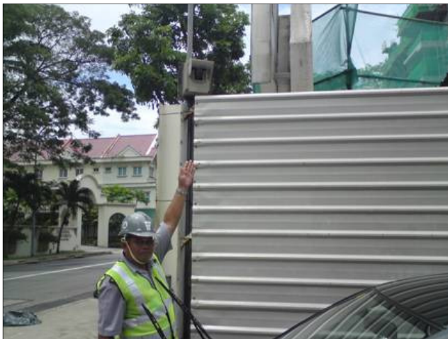
Photo 2.7e: CCTV can be used by the builder to enhance the security on site and minimize security concerns of neighbouring residents.
